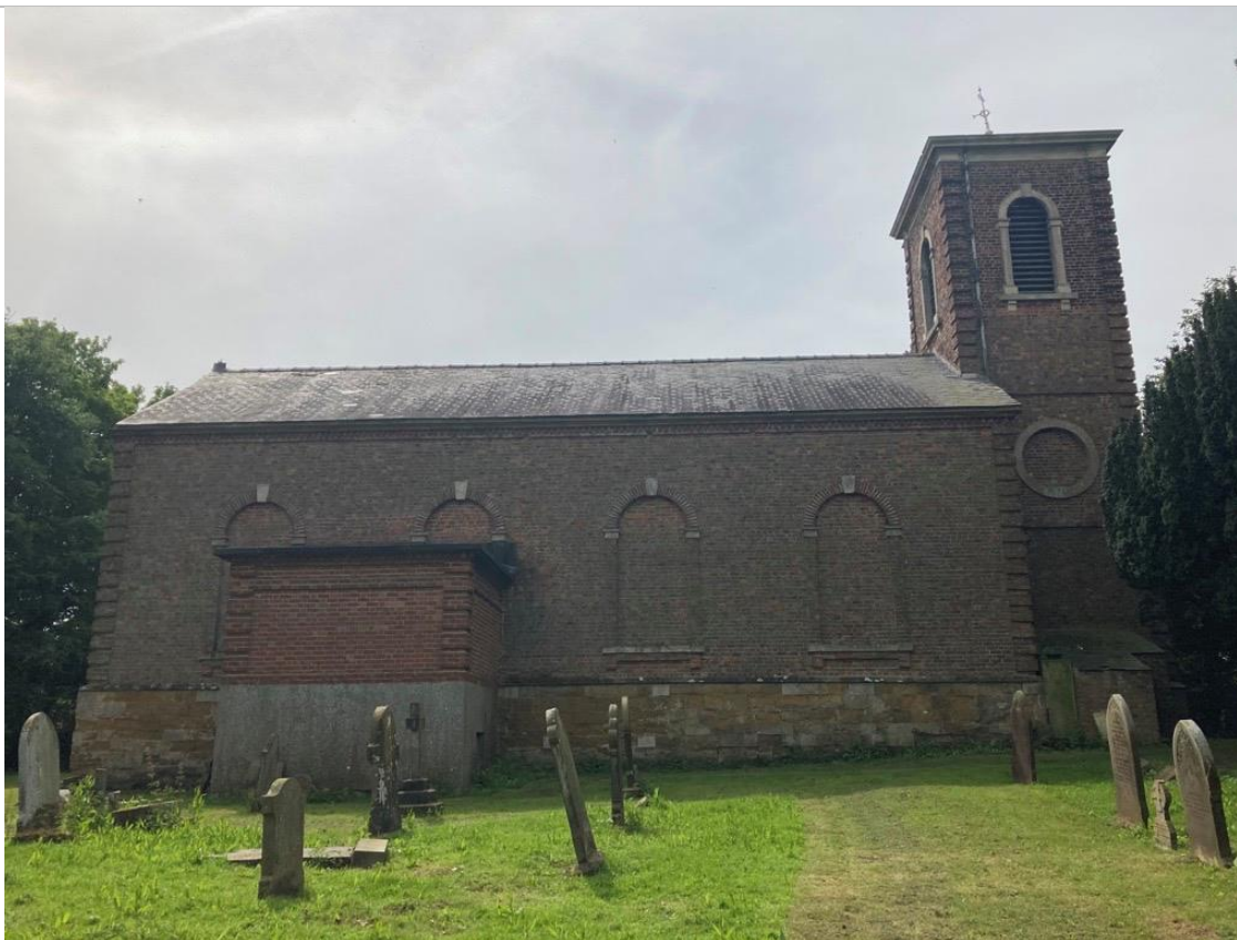
Plate 10 Church of St Peter and St Paul, Church Lane, Stallingborough [178]
